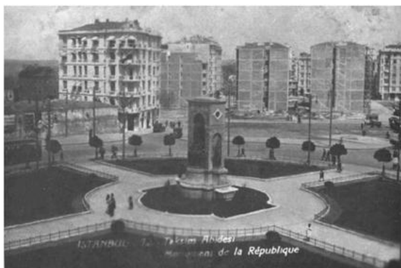
Figure 7: Construction of the monument (Gülersoy, 1986, 32).
