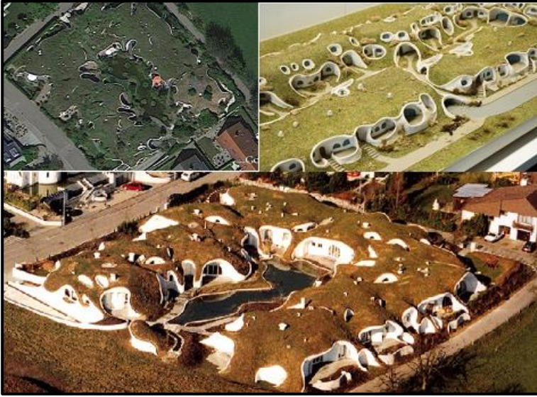
Figure 1. Earth House, Peter Vetsch (URL-1)
